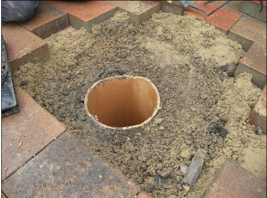
Figure 14 - Chamber reduced to formation level
