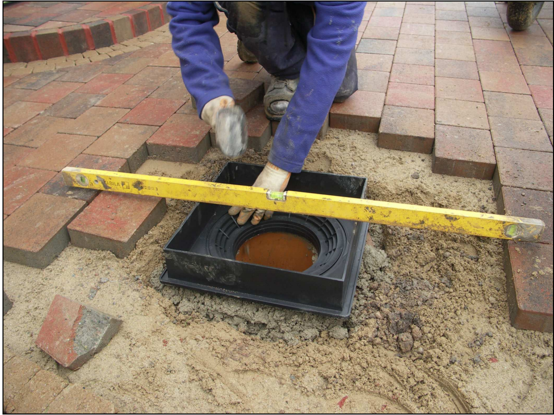
Figure 7 - Place frame and set to level
