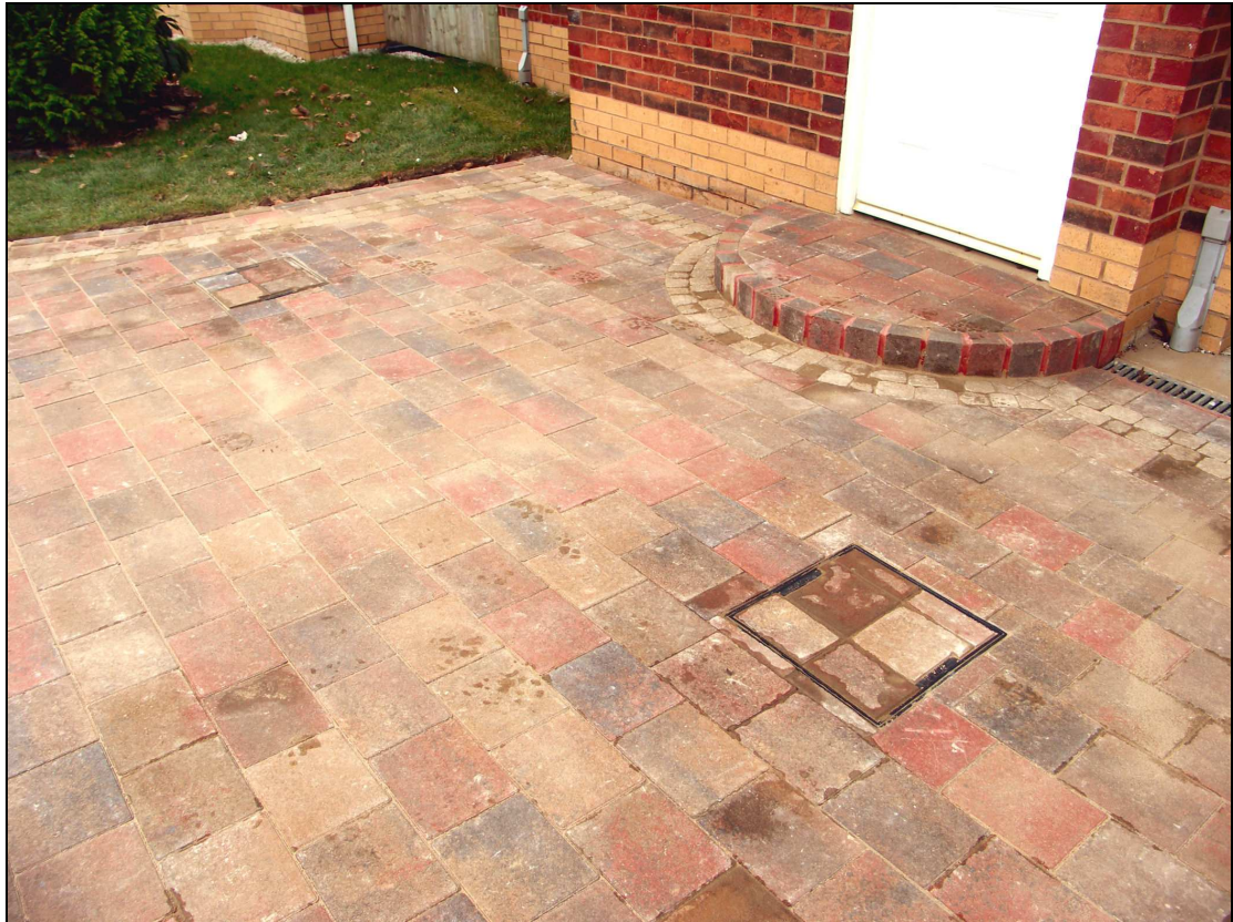
Figure 20 - Two covers completed and in place
