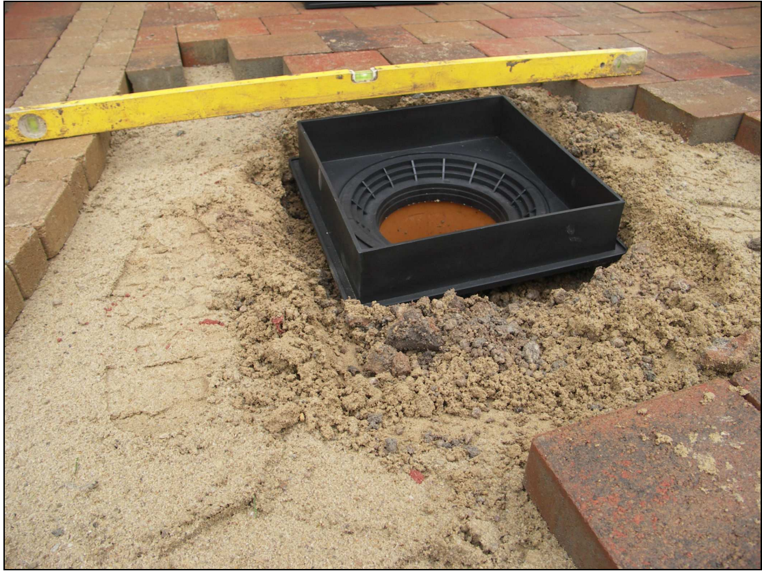
Figure 3 - Testing level of cover
