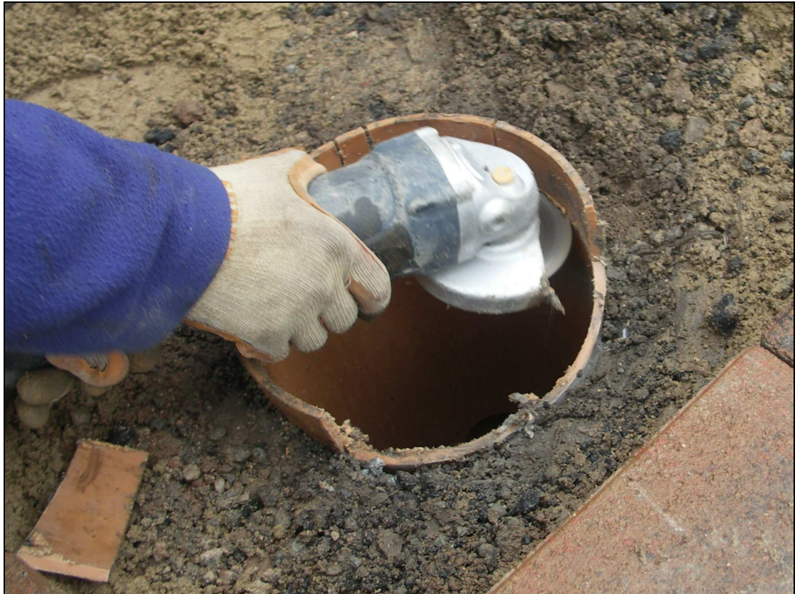
Figure 13 - Making horizontal cuts in chamber wall
