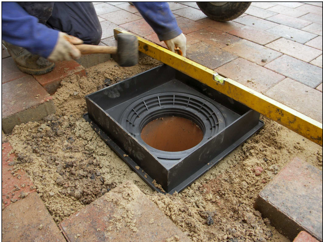
Figure 16 - Tapping down frame to required level
