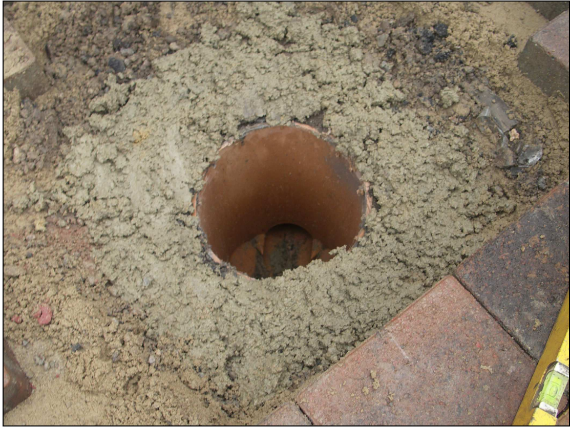
Figure 15 - Mortar bed for Frame
