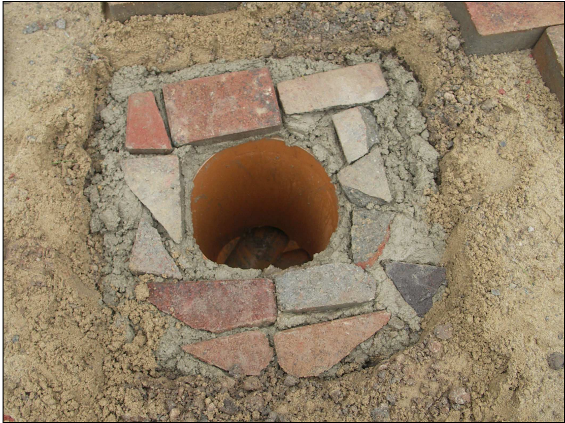
Figure 5 - Concrete shims laid onto mortar bed
