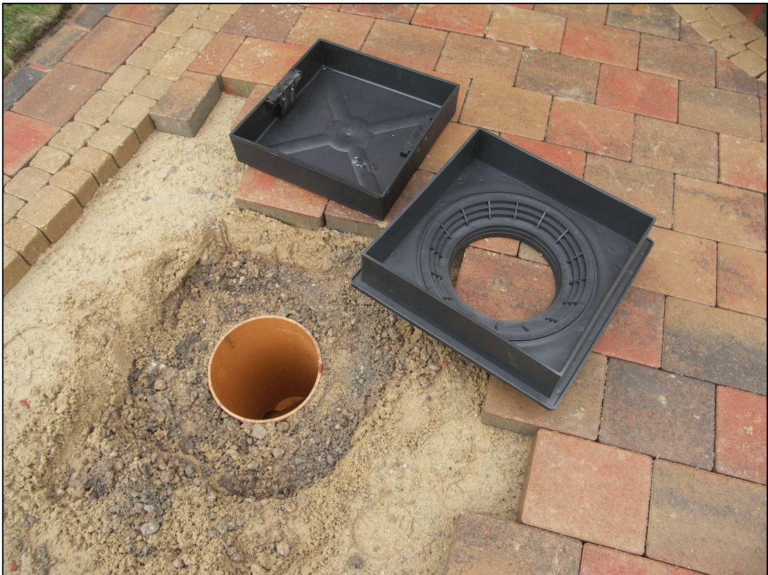
Figure 2 - Old cover removed and 300SR brought in
